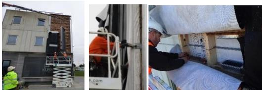
Figure 4. Installing the panels. Fixing the connector. Joining and fitting services
