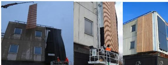
Figure 5. Finishing placement and fixation. Final enclosure and perimeter finishing.
